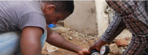
(pipe-laying, laying of the general water meter, stop, meter clusters, impounding). The pressure tests are being finalized, as well as the construction of the meter columns. Afterwards will come the disinfection of the network. The teams are in the middle of a prospection phase in the neighborhood to inform the inhabitants and in a recruitment phase of collectors, essential element of Eau et Vie's chain.
