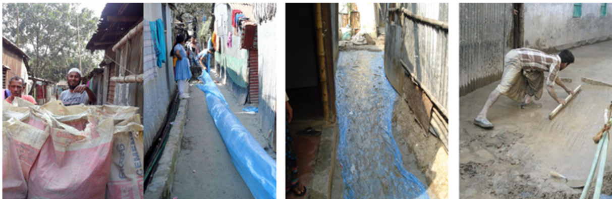
Gutter installation for wastewater draining and alley cement.
