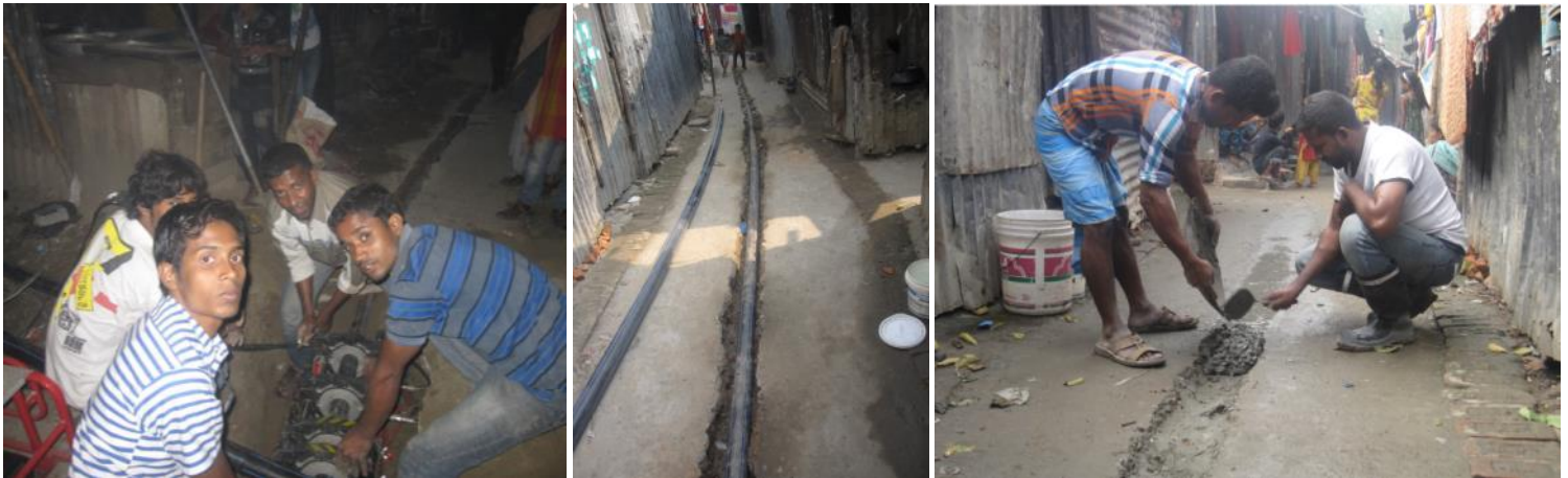
Bhashantek (Bangladesh): Installing the main pipeline – HDPE pipes – Cementing the alleyways
