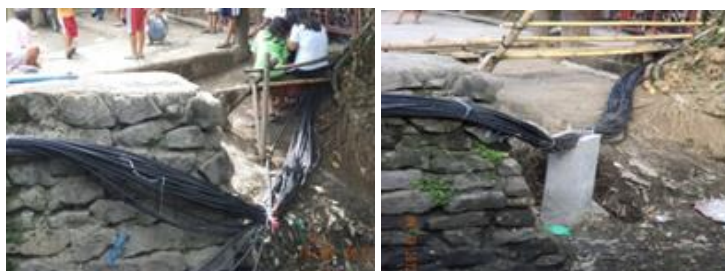
Manggahan: Repairs following a typhoon in September
