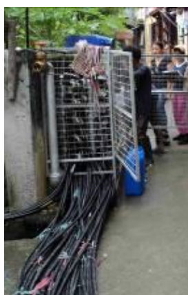
Connections before cementing
