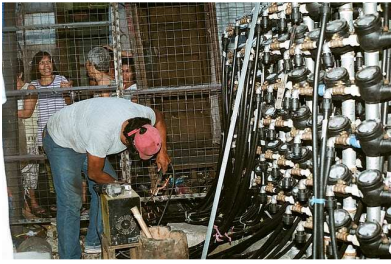
Meters were grouped together in a cluster and the installation was secured
