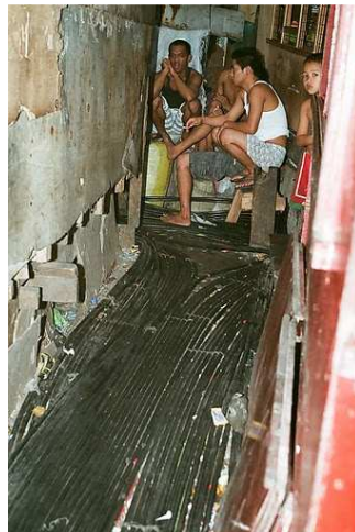
Pipes were connected directly to the homes
