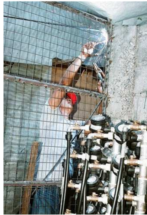
Meters were grouped together in a cluster and the installation was secured
