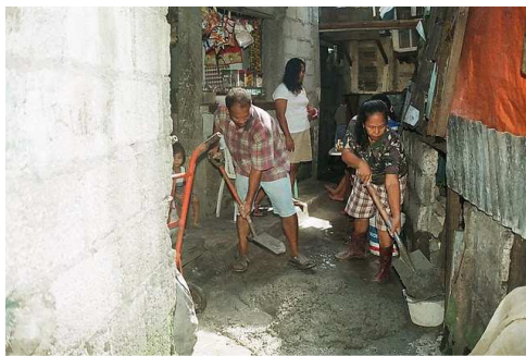
Building finishing and covering up of the paths with cement
